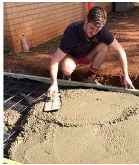
(Left) Chad Hartin floating a concrete slab (Peak Hill) (Right) Sam Jackson with his Carry All Toolbox (Tottenham)
